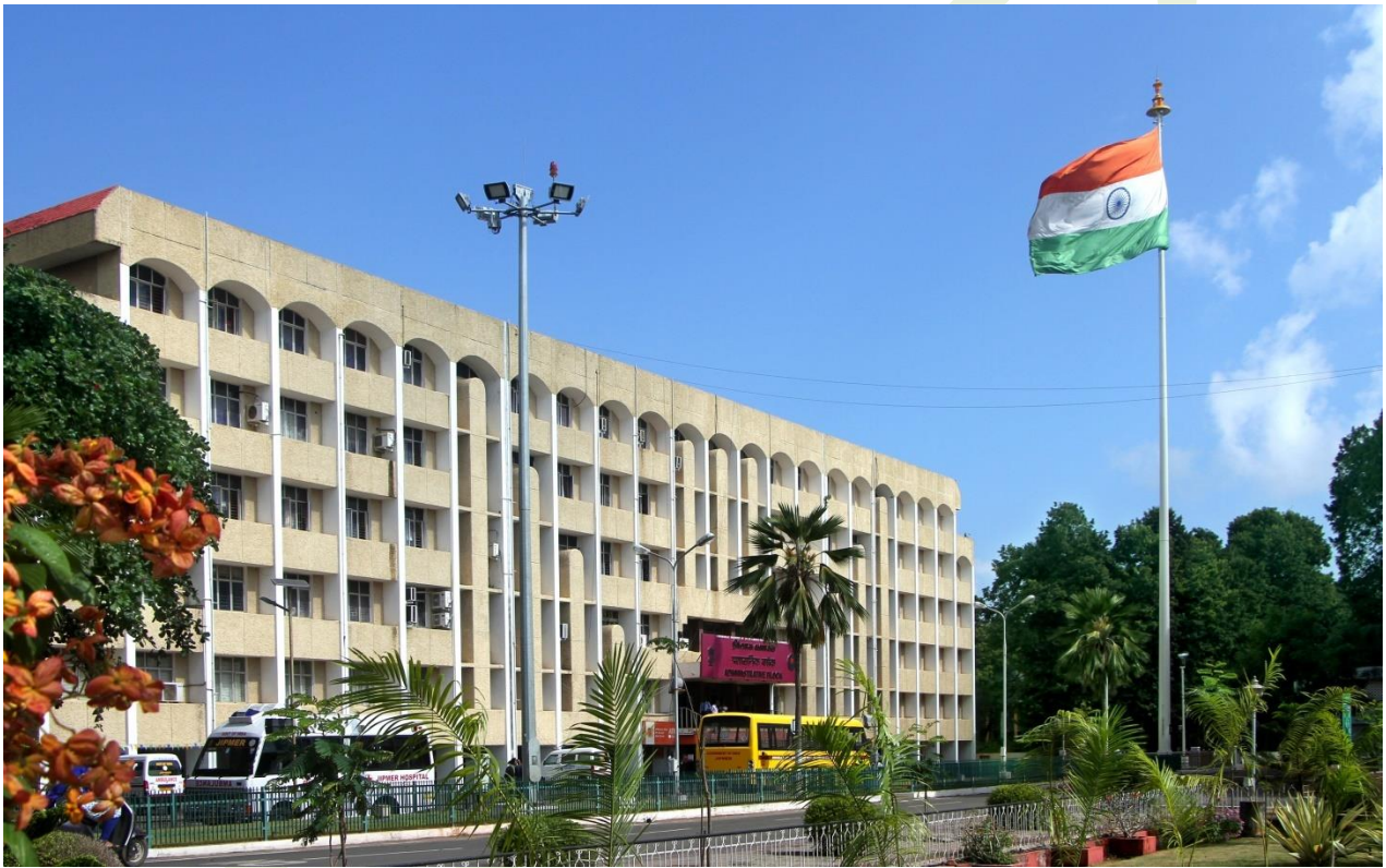
Administrative Block, JIPMER Puducherry
